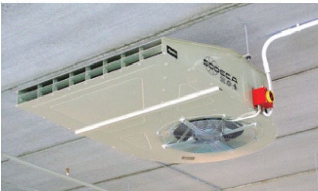
CI installed in car park
