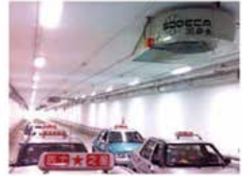
Tunnel Projects Shanghai, China
